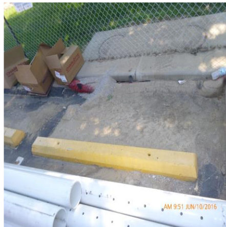
REMOVE SEDIMENT BUILDUP AT DCI 23K2-0374D
