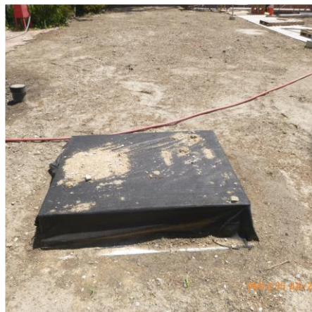
INLET PROTECTION IN PLACE
