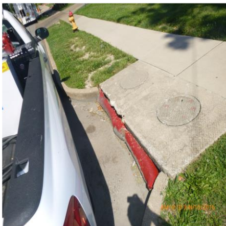
CURB INLET PROTECTION ON GARDEN AVENUE
