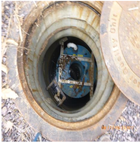
INSIDE VIEW OF DOWNSTREAM DEFENDER
