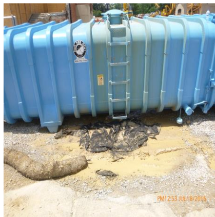
WATER COLLECTION TANK & INLET 1
