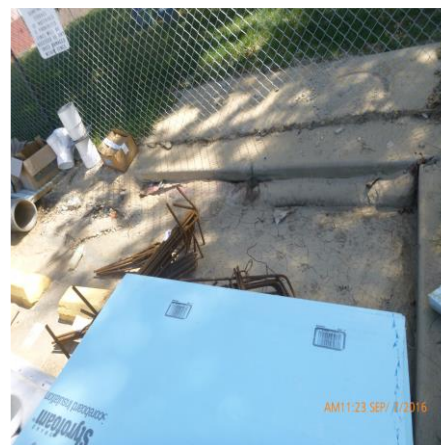
REMOVE SEDIMENT IN FROM OF INLET
