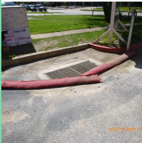
INLET PROTECTION IN PLACE
