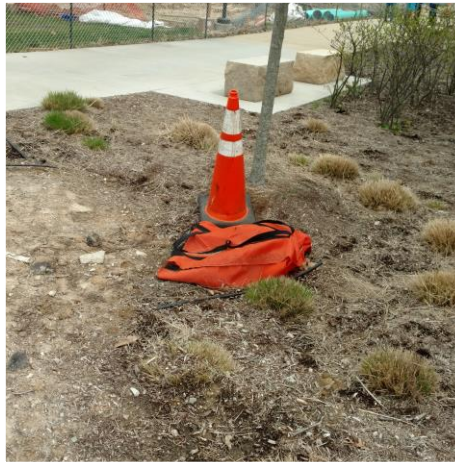
INLET PROTECTION IN PLACE
