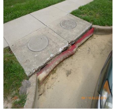
REMOVE SEDIMENT IN FRONT OF INLET PROTECTION
