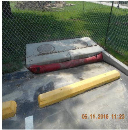
CURB INLET PROTECTION IN PLACE AT DCI 23K2-0374D
