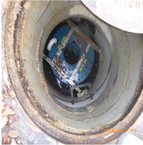
LOOKING INSIDE THE DOWNSTREAM DEFENDER
