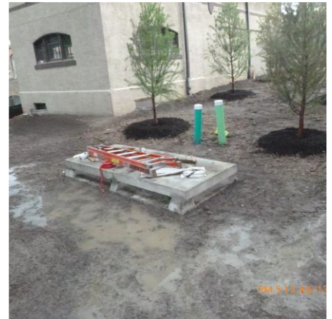
ADD PROTECTION TO AREA INLET # 6
