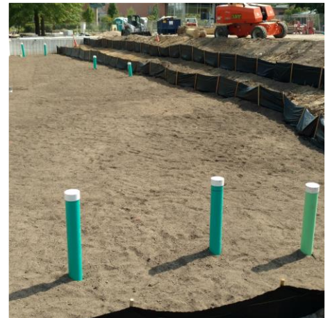
SILT FENCE IN PLACE AROUND RAIN GARDEN # 1
