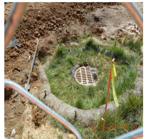
MONITOR CONDITION OF INLET PROTECTION
