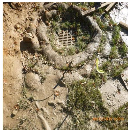
INLET PROTECTION IN PLACE
