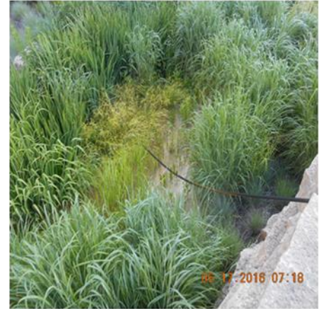
SEDIMENT BUILDUP TO THE EAST OF HDS OUTLET PIPE
