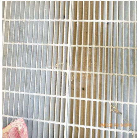
REMOVE AND REPLACE FILTER FABRIC
