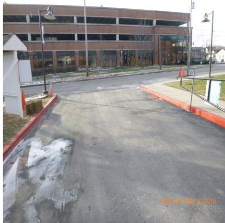
LOOKING AT SITE ENTRANCE FROM GARDEN AVENUE
