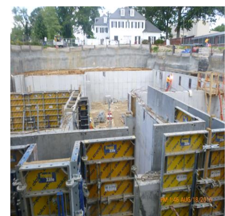
LOOKING NORTH AT MIDDLE OF CONSTRUCTION SITE
