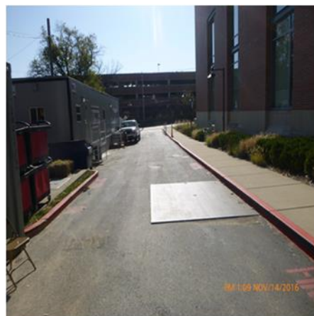
LOOKING SOUTH AT CONSTRUCTION SITE ENTRANCE
