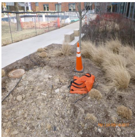
INLET PROTECTION IN PLACE
