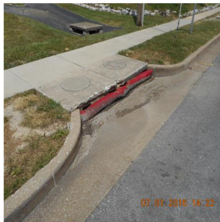
REMOVE SEDIMENT IN FRONT OF INLET PROTECTION
