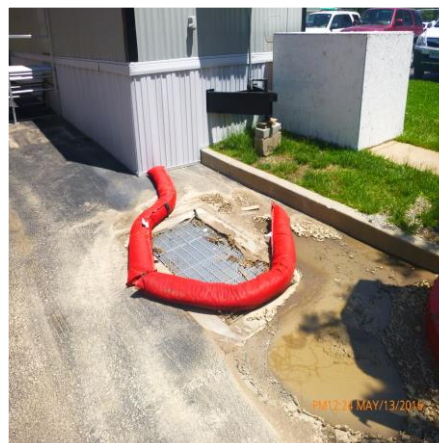
INLET PROTECTION IN PLACE AT SE CORNER OF EAST ACADEMIC BUILDING
