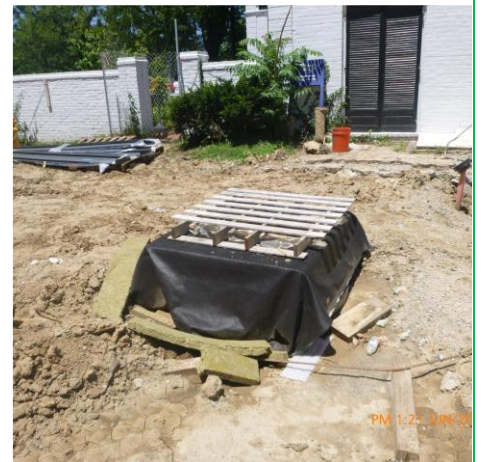
INLET PROTECTION IN PLACE
