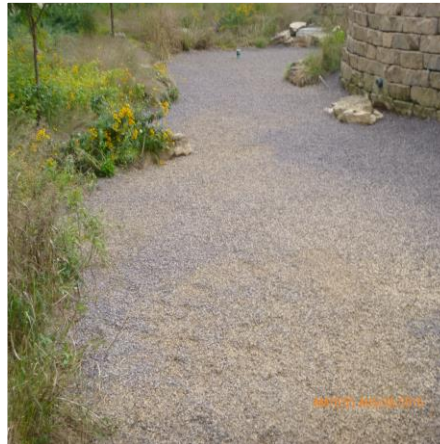
LOOKING AT MINOR SEDIMENT ON TOP OF ROCK IN RAIN GARDEN
