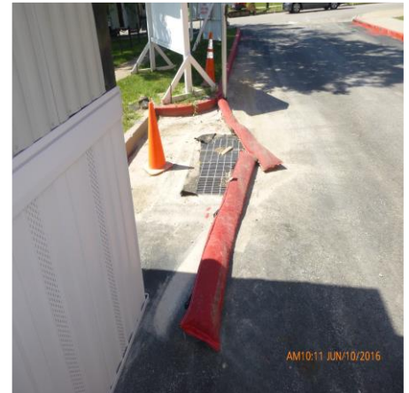
PIN OR WEIGH DOWN INLET PROTECTION 23K2-0394D
