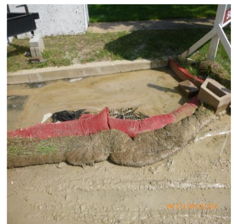
REPLACE FILTER FABRIC AS NEEDED
