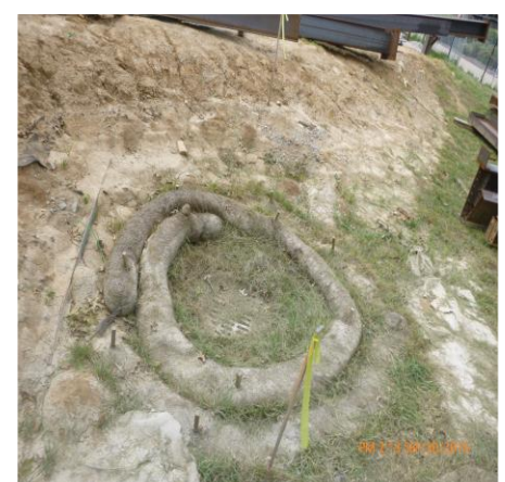
INLET PROTECTION IN PLACE
