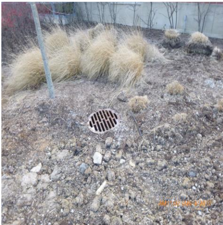
MONITOR SEDIMENT AT CURB INLET (PARKING LOT)
