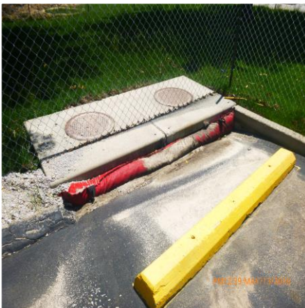
INLET PROTECTION IN PLACE AT DCI 23K2-0374D
