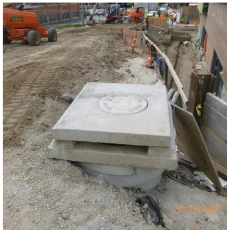
ADD PROTECTION TO AREA INLET # 3
