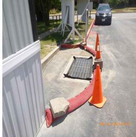
INLET PROTECTION IN GOOD CONDITION
