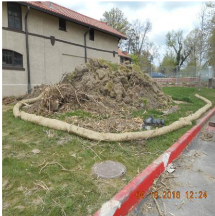
VIEW OF SEDIMENT BARRIER AROUND SOIL STOCKPILE
