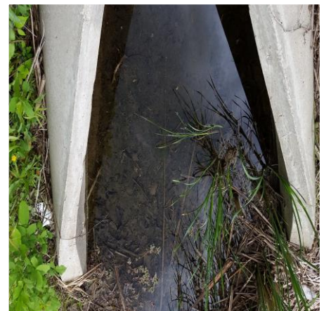
LOOKING AT EAST INLET PIPE INTO LAKE SOUTH OF PROJECT SITE
