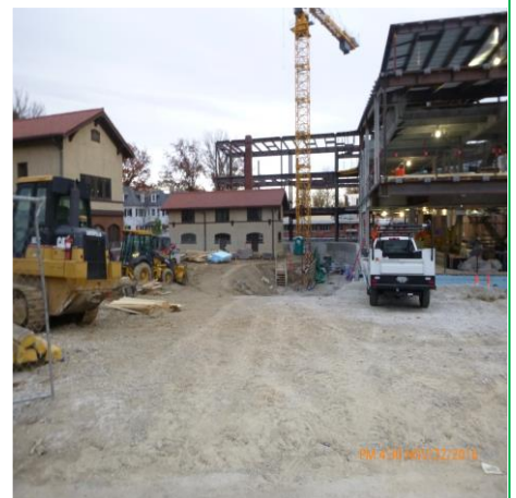
LOOKING EAST AT MIDDLE OF CONSTRUCTION SITE
