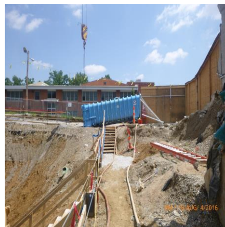
DEWATERING TANK BY INLET # 1
