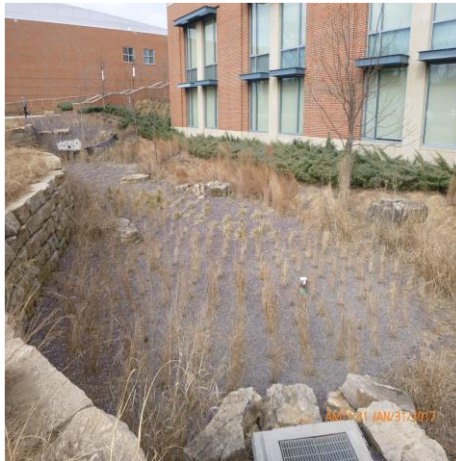
REMOVE SEDIMENT AT INLET (GARDEN AVE) AND AREA OF GRASS
