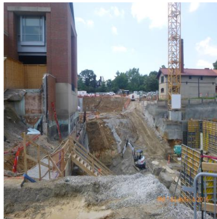
LOOKING WEST AT MIDDLE OF CONSTRUCTION SITE
