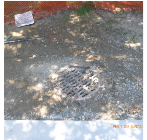
INLET PROTECTION IN PLACE
