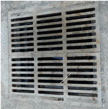
VIEW OF DBL GRATE INLET # 1
