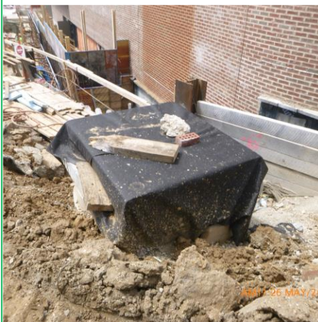
INLET PROTECTION IN PLACE
