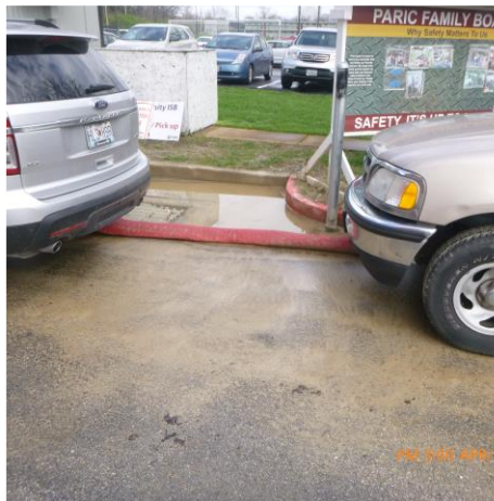
INLET PROTECTION IN PLACE
