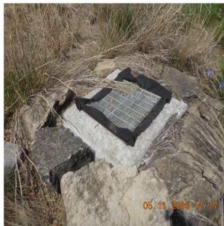
FILTER FABRIC UNDER GRATES IN RAIN GARDEN GI 23K2-0391D
