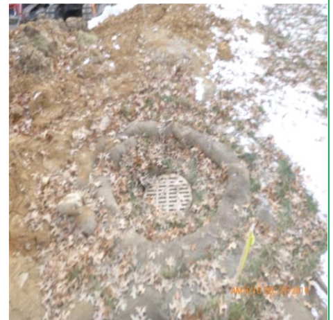
INLET PROTECTION IN PLACE
