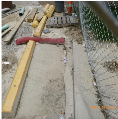
MONITOR SEDIMENT AT CURB INLET (PARKING LOT)
