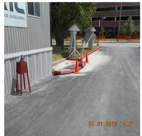
VIEW OF INLET PROTECTION AT FOUR GRATE INLET
