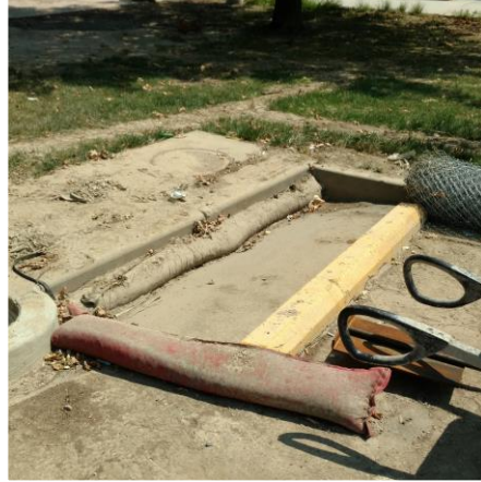
MONITOR SEDIMENT BUILDUP AT CURB INLET (PARKING LOT)
