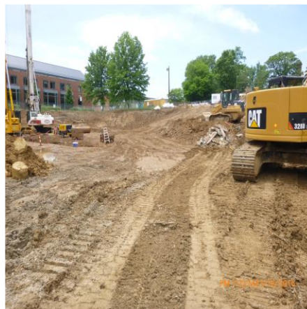
LOOKING WEST AT MIDDLE OF CONSTRUCTION SITE
