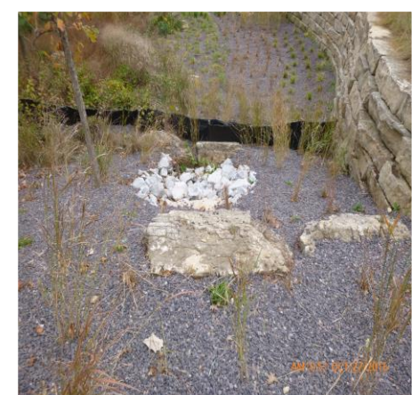
SILT FENCE IN PLACE IN RAIN GARDEN
