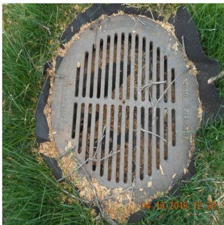
LOOKING AT SEDIMENT PROTECTION IN GI 23K2-0444D
