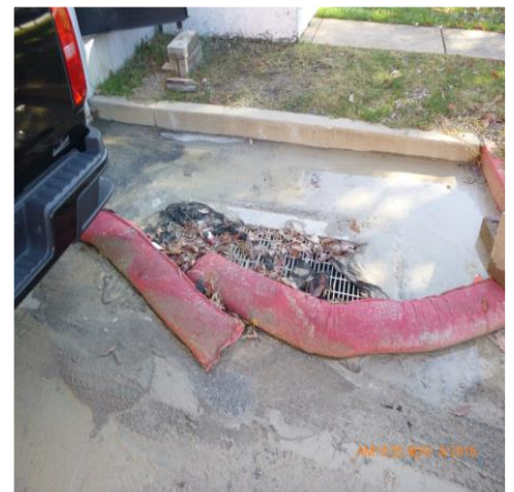
REPLACE FILTER FABRIC AS NEEDED
