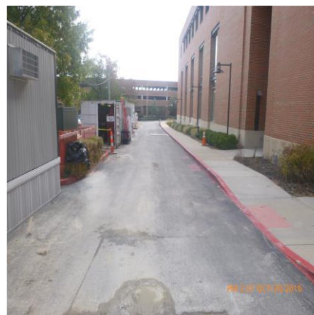
LOOKING SOUTH AT CONSTRUCTION DRIVEWAY ENTRANCE
