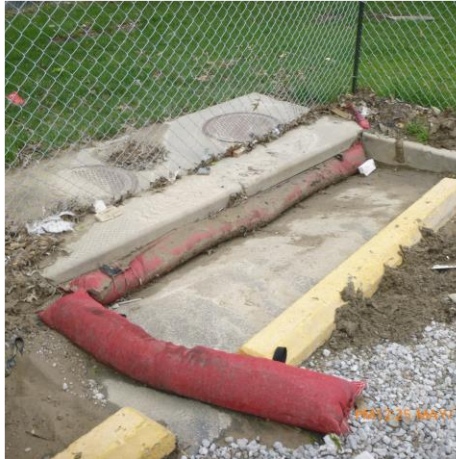
ADDITIONAL SILT SOCK ADDED TO CURB INLET (PARKING LOT)
