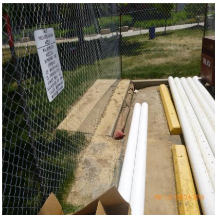
MONITOR CONDITION OF INLET PROTECTION
