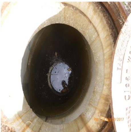
INLET PROTECTION IN PLACE (GARDEN AVENUE)
