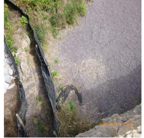
SILT FENCE REPAIRED AT RAIN GARDEN
