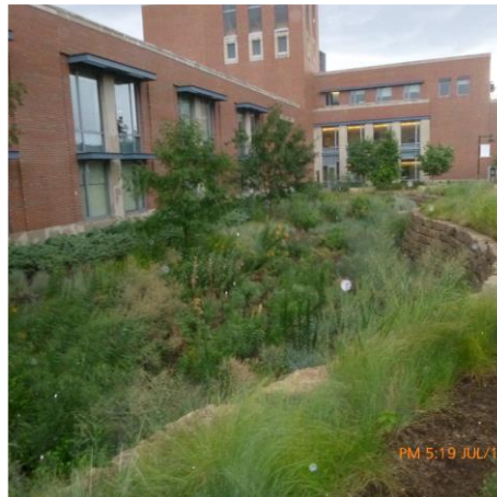
VIEW OF RAIN GARDEN A
