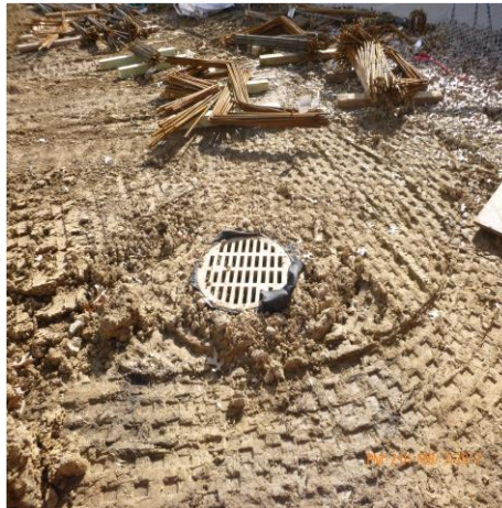
FILTER FABRIC IN PLACE INLET # 23K2-040D
