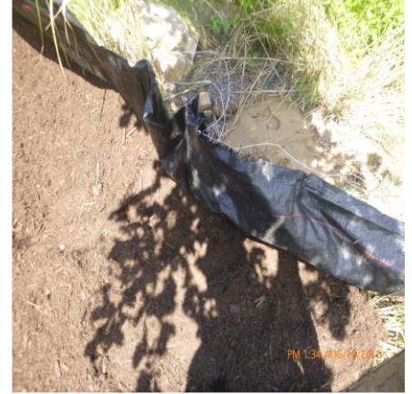
REPAIR UNDERMINED SILT FENCING BELOW DOWNSTREAM DEFENDER
