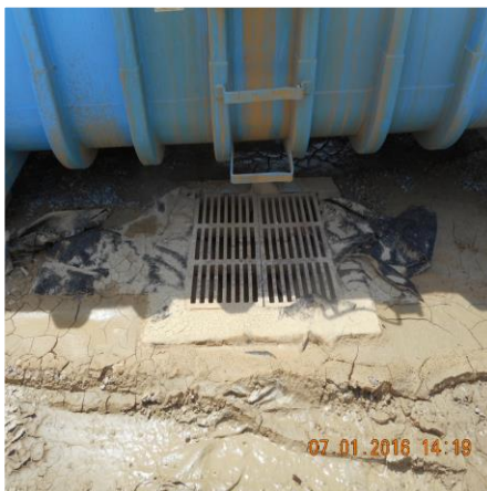
LOOKING AT DEWATERING TANK AND INLET PROTECTION
