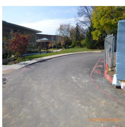
LOOKING WEST AT CONSTRUCTION SITE ENTRANCE
