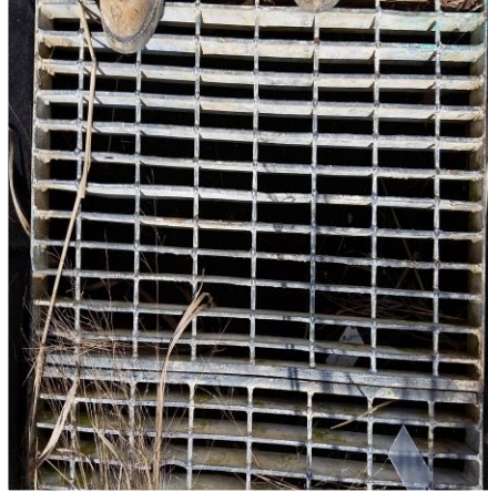
LOOKING AT SEDIMENT PROTECTION IN GI 23K2-0391D
