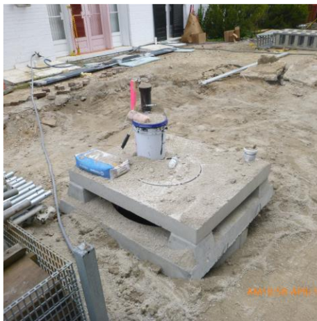
ADD PROTECTION TO AREA INLET # 4
