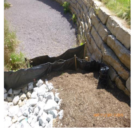
REINSTALL SILT FENCING BELOW DOWNSTREAM DEFENDER
