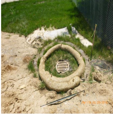
INLET PROTECTION IN PLACE
