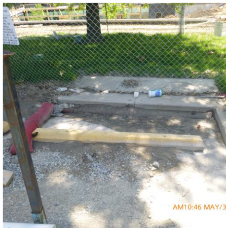
REMOVE SEDIMENT AROUND CURB INLET
