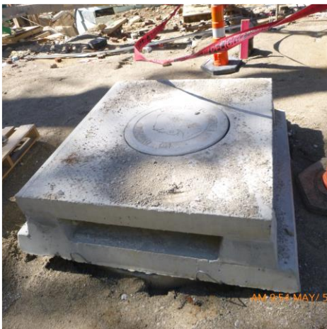
ADD PROTECTION TO AREA INLET # 4
