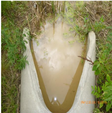
REMOVE SEDIMENT IN FRONT OF INLET PROTECTION
