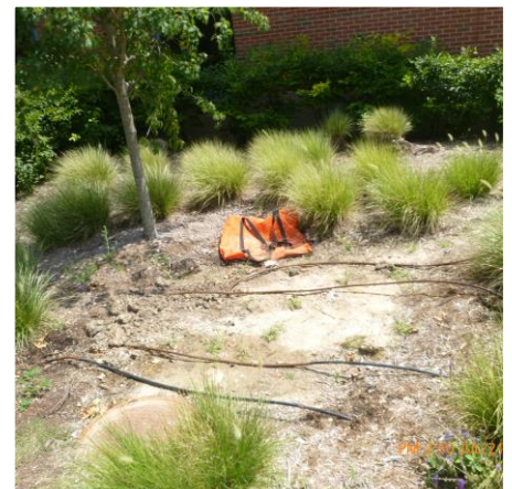
INLET PROTECTION IN PLACE
