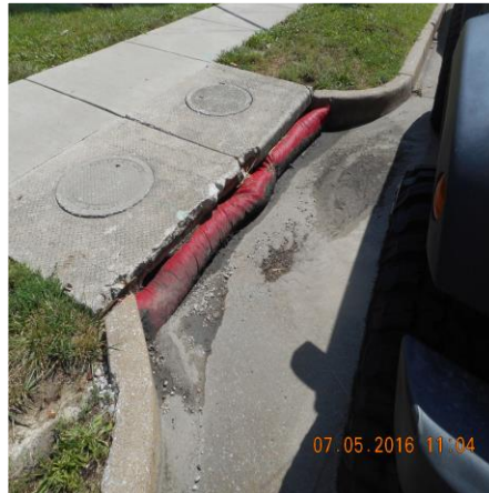
REMOVE SEDIMENT IN FRONT OF INLET PROTECTION
