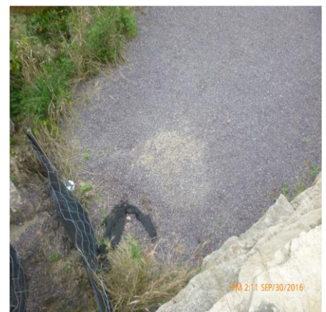
MONITOR SEDIMENT ENCROACHMENT IN RAIN GARDEN
