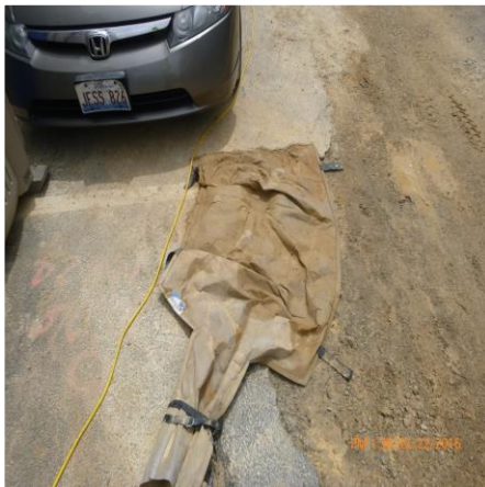
FILTER BAG AFTER COLLECTING SEDIMENT BEFORE DISCHARGING
