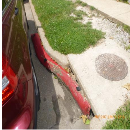
CURB INLET PROTECTION ON GARDEN AVENUE
