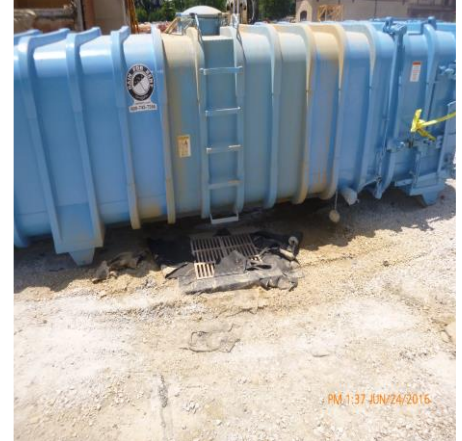
DEWATERING TANK AND INLET PROTECTION IN GOOD CONDITION
