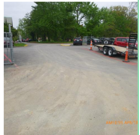
LOOKING WEST AT SITE ENTRANCE (PARKING LOT)
