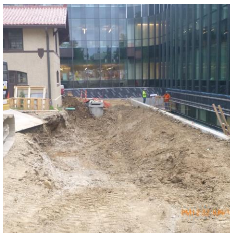
EXCAVATION OF RAIN GARDEN STARTING
