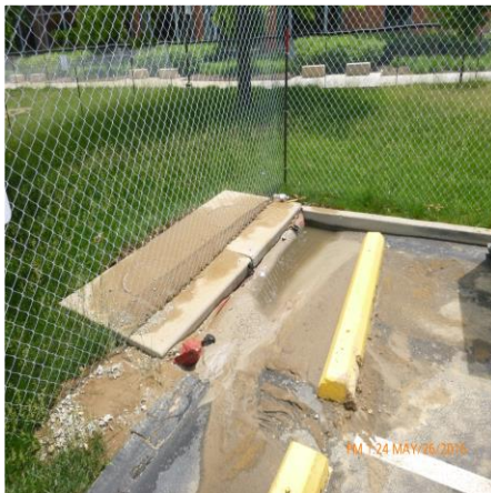
REMOVE SEDIMENT BUILDUP AT DCI 23K2-0374D
