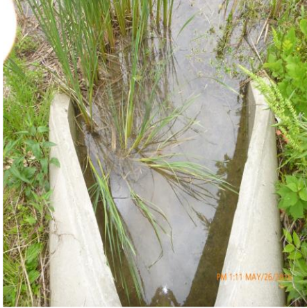
REMOVE SEDIMENT BUILDUP AT DCI 23K2-0374D
