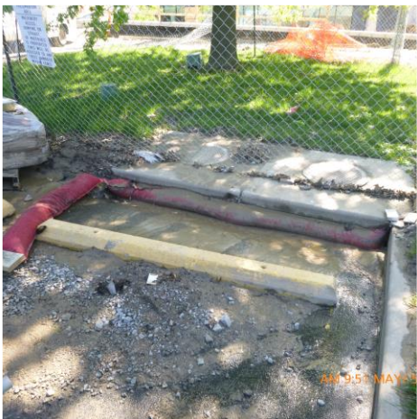
MONITOR SEDIMENT AT CURB INLET (PARKING LOT)
