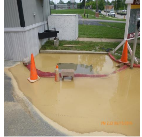
REPLACE FILTER FABRIC TO REMOVE STANDING WATER
