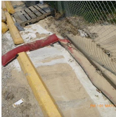
MONITOR SEDIMENT AT CURB INLET (PARKING LOT)
