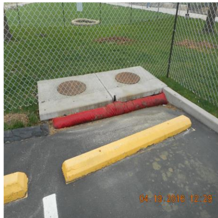
BIG RED INLET PROTECTION IN PLACE AT DCI 23K2-0374D
