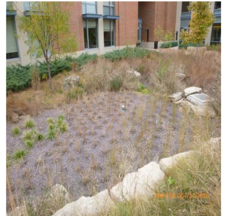
VIEW OF NEW PLANTS IN RAIN GARDEN A
