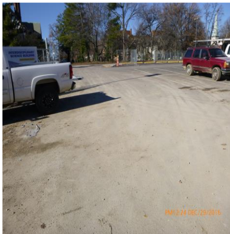
MONITOR SEDIMENT AT PARKING LOT ENTRANCE
