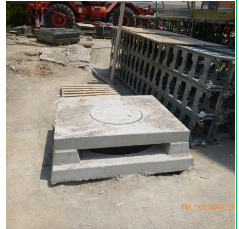
ADD PROTECTION TO AREA INLET # 4
