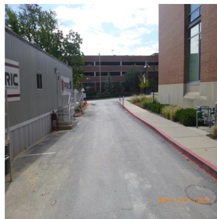
LOOKING SOUTH AT CONSTRUCTION DRIVEWAY ENTRANCE
