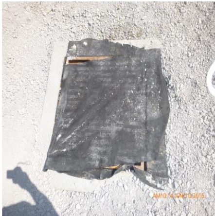
FILTER FABRIC COVERING INLET # 1
