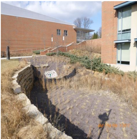
REMOVE SEDIMENT AND DEBRIS FROM INLET (PARKING LOT)
