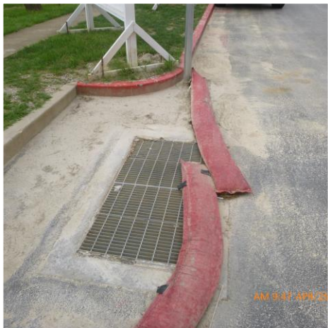
INLET PROTECTION IN PLACE
