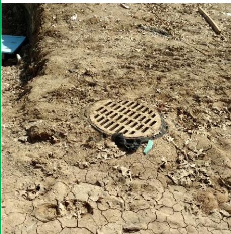
INLET PROTECTION IN PLACE
