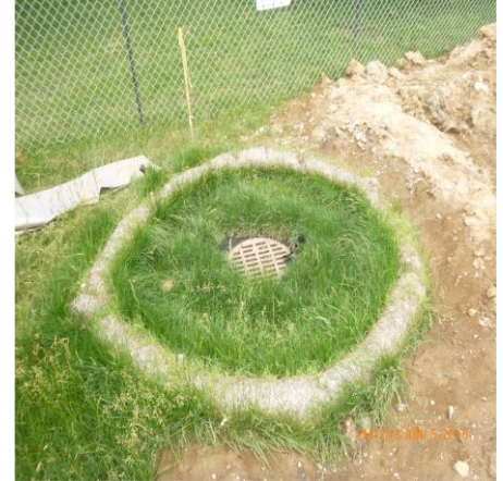
SILT SOCK AND FILTER FABRIC PROTECTING GI 23K2-0406D
