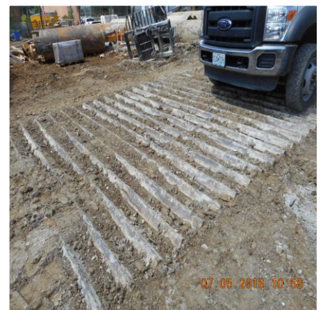
MONITOR CONDITION OF EXIT RAMP RUMBLE STRIPS
