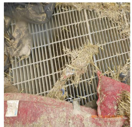
REPLACE FILTER FABRIC AS NEEDED
