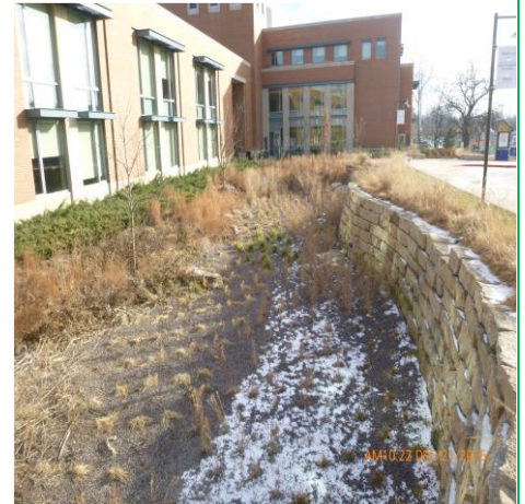
VIEW OF RAIN GARDEN A
