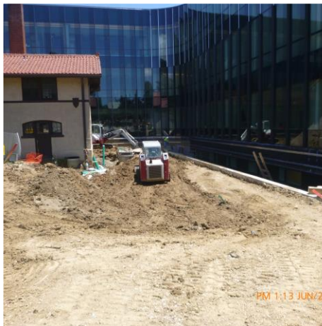
EXCAVATION OF RAIN GARDEN STARTING
