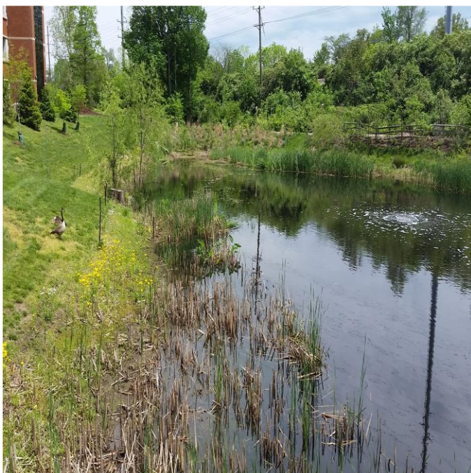
LOOKING EAST TOWARD INLET PIPE FES
