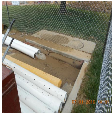
REMOVE SEDIMENT IN FRONT OF INLET PROTECTION
