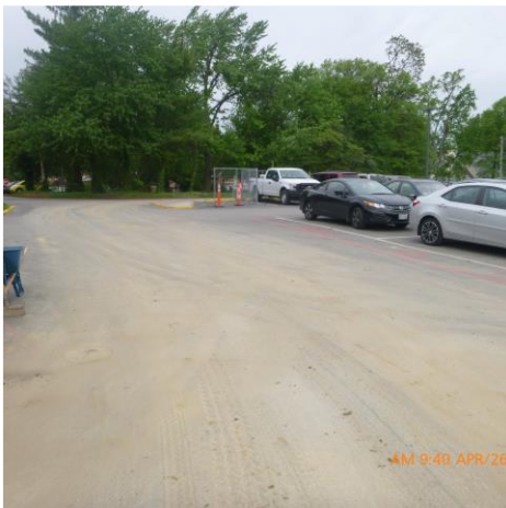
MONITOR SEDIMENT AT SITE ENTRANCE (PARKING LOT)
