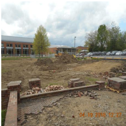
LOOKING SOUTH ACROSS LAND DISTURBED TO DATE
