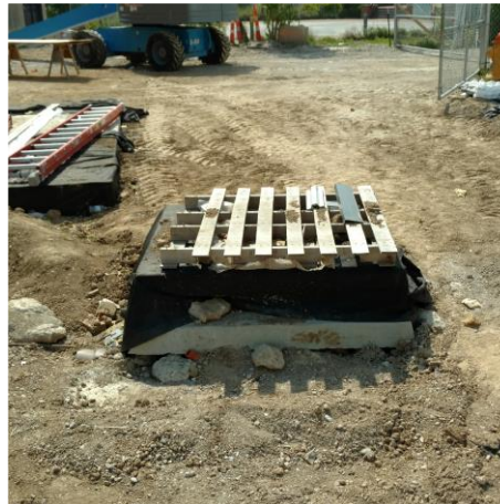
INLET PROTECTION IN PLACE
