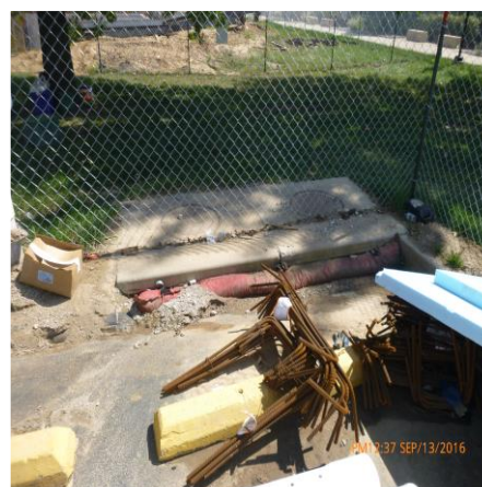
REMOVE SEDIMENT IN FROM OF INLET
