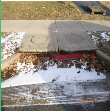
MONITOR SEDIMENT AT CURB INLET (GARDEN AVENUE)
