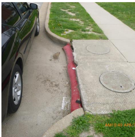
INLET PROTECTION IN PLACE (GARDEN AVENUE)
