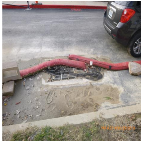
REPLACE FILTER FABRIC AS NEEDED
