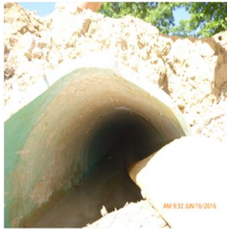
VIEW INTO STORM SEWER CARRYING TURBID WATER TO HDS
