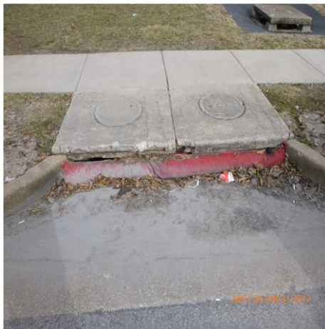
REMOVE SEDIMENT AT INLET (GARDEN AVE) AND AREA OF GRASS
