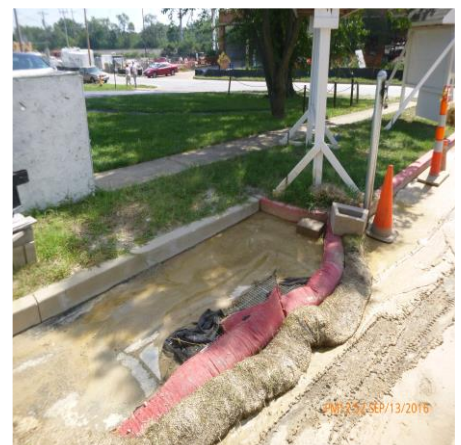
REPLACE FILTER FABRIC AS NEEDED
