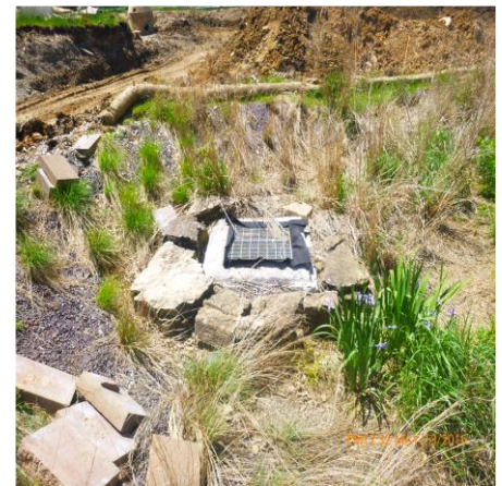
FILTER FABRIC UNDER GRATES IN RAIN GARDEN GI 23K2-0391D
