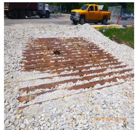
LOOKING WEST AT TRUCK WASH DOWN AREA
