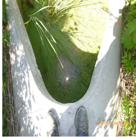
REMOVE SEDIMENT BUILDUP AT DCI 23K2-0374D
