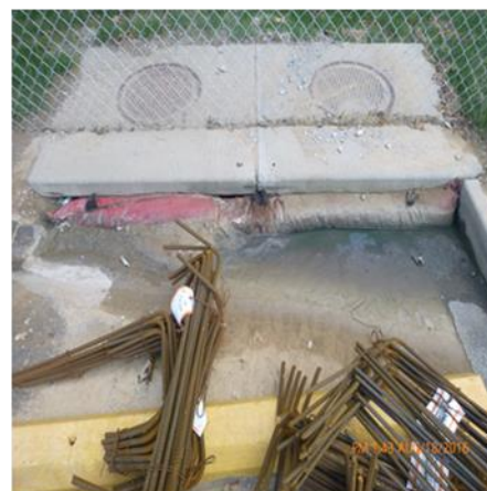
REMOVE SEDIMENT IN FROM OF INLET
