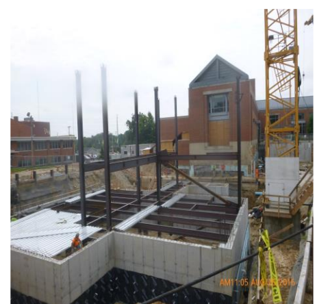
LOOKING SOUTH AT MIDDLE OF CONSTRUCTION SITE
