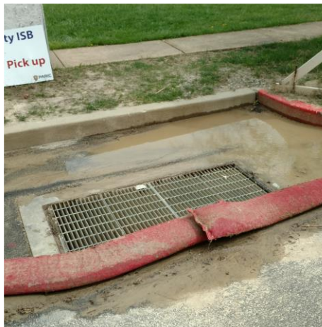
INLET PROTECTION IN PLACE
