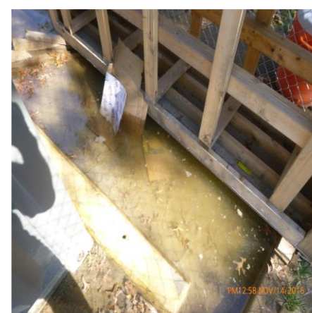
REMOVE SEDIMENT FROM IN FRONT OF CURB INLET
