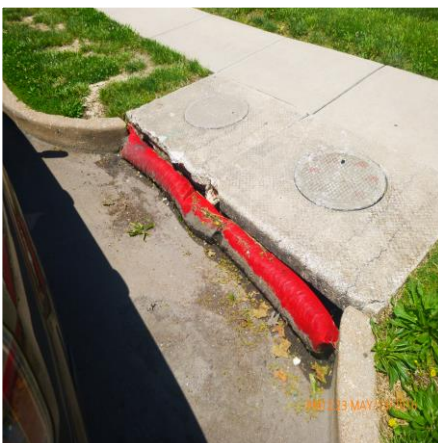
INLET PROTECTION IN PLACE AT DCI ON GARDEN AVENUE
