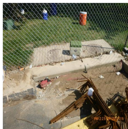
REMOVE SEDIMENT IN FROM OF INLET
