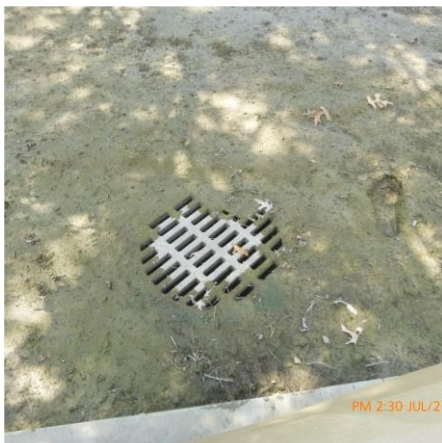
INLET PROTECTION IN PLACE
