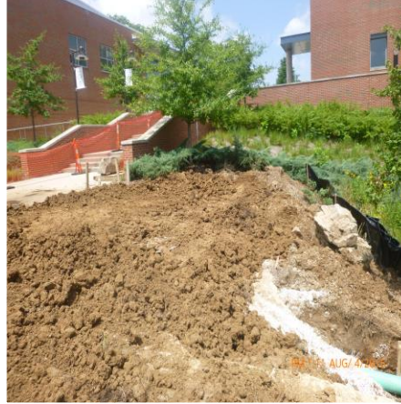
LOOKING AT THE DOWNSTREAM DEFENDER PROJECT
