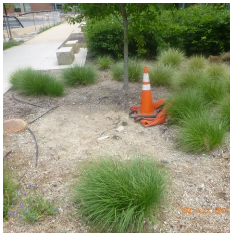
INLET PROTECTION IN PLACE
