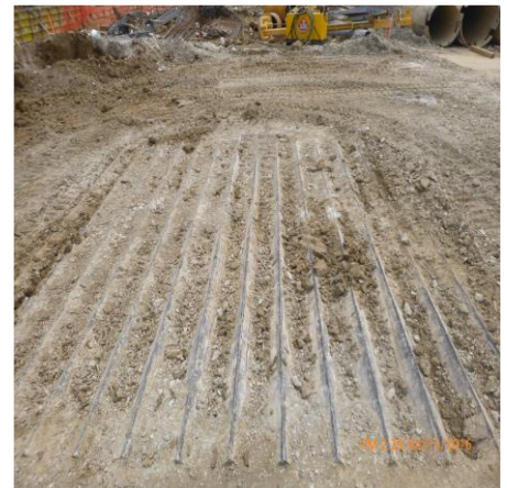
MONITOR CONDITION OF EXIT RAMP RUMBLE STRIPS
