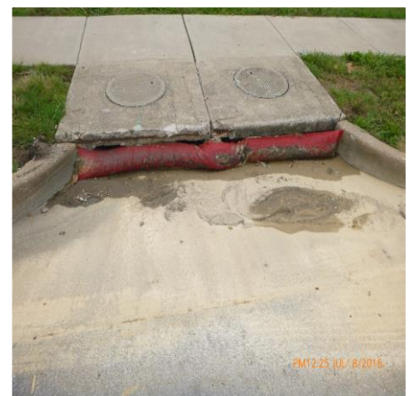
INLET PROTECTION IN PLACE AT GARDEN AVENUE
