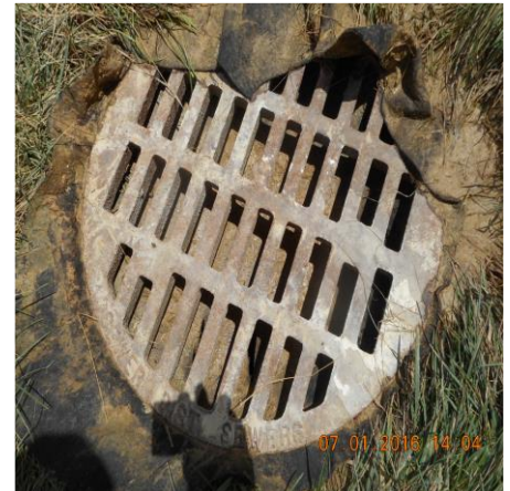
REMOVE AND REPLACE FILTER FABRIC AT INLETS AS NEEDED
