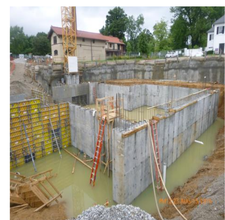
LOOKING NW AT MIDDLE OF CONSTRUCTION SITE
