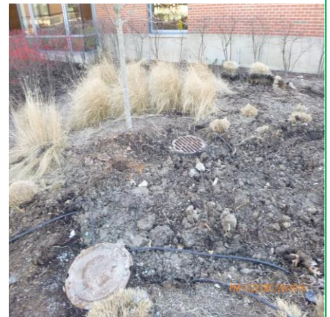
ADD INLET PROTECTION TO 23K2-0407D
