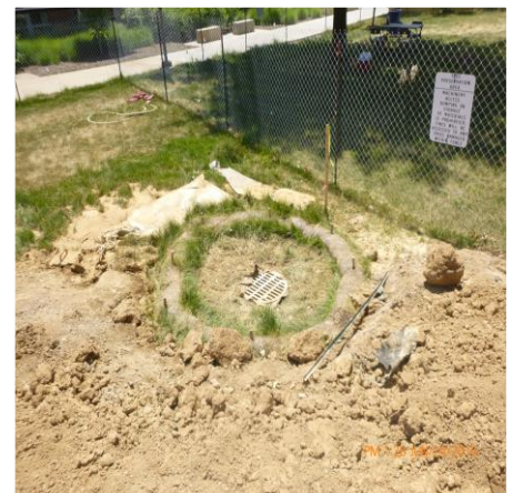
MONITOR CONDITION OF INLET PROTECTION
