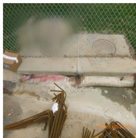
REMOVE SEDIMENT IN FROM OF INLET
