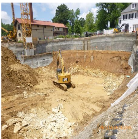
LOOKING NORTHWEST AT MIDDLE OF CONSTRUCTION SITE
