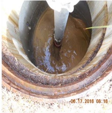
VIEW INTO HDS WITH SEDIMENT DEPTH OF 6'-11"
