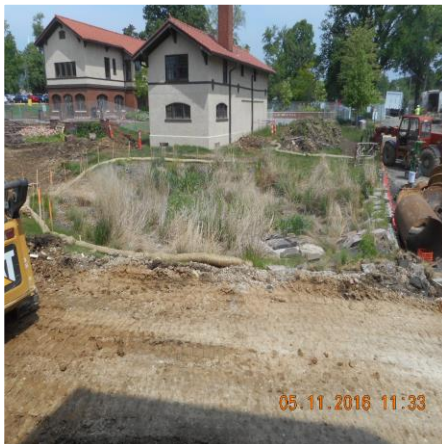
VIEW OF SEDIMENT PROTECTION AROUND EXISTING RAIN GARDEN
