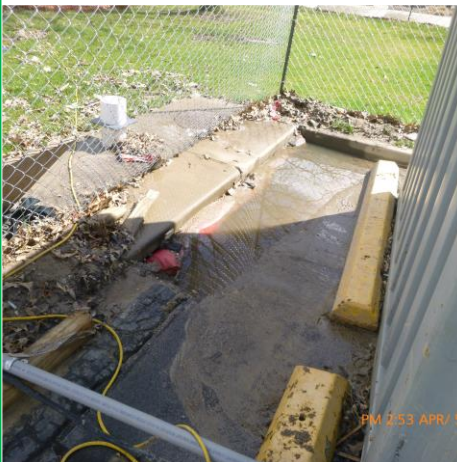
MONITOR SEDIMENT AT CURB INLET (PARKING LOT)
