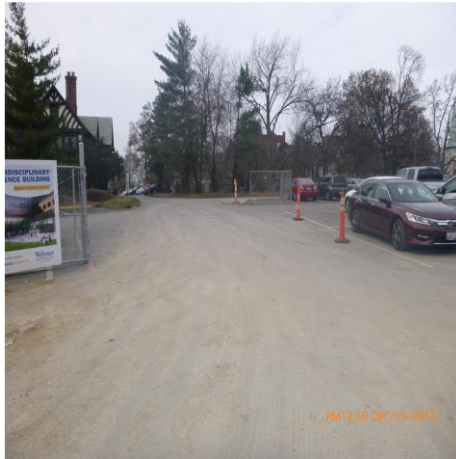
MONITOR SEDIMENT AT PARKING LOT ENTRANCE
