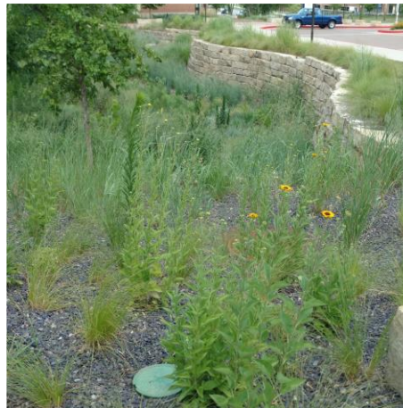
VIEW OF RAIN GARDEN A
