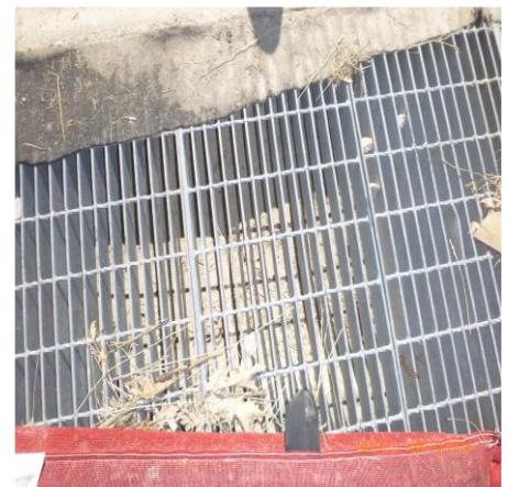
FILTER FABRIC IN PLACE AT GI 23K2-0394D
