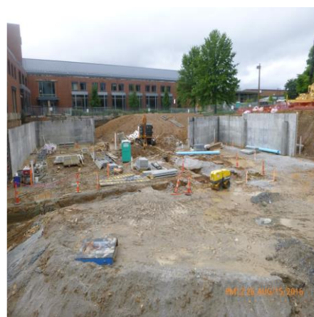
LOOKING SW AT MIDDLE OF THE CONSTRUCTION SITE
