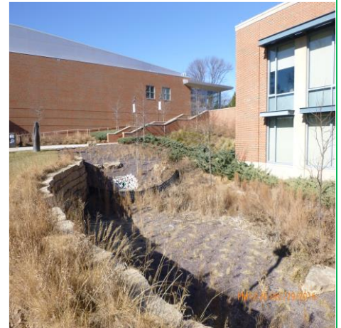
VIEW OF RAIN GARDEN A
