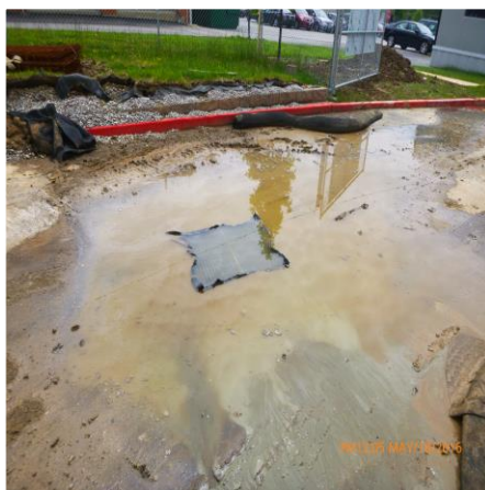
REMOVE AND REPLACE FILTER FABRIC IN GI 23K2-0392D
