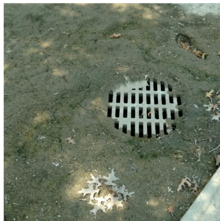
INLET PROTECTION IN PLACE
