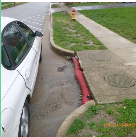
INLET PROTECTION IN PLACE
