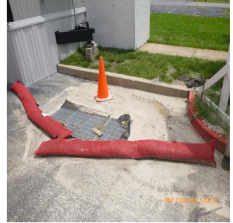
PIN OR WEIGH DOWN INLET PROTECTION 23K2-0394D
