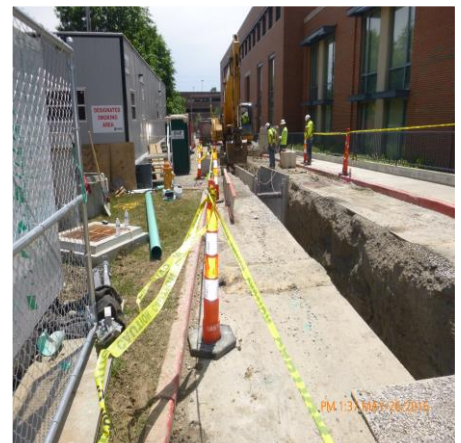
STORM SEWER INSTALLATION EAST OF EAB
