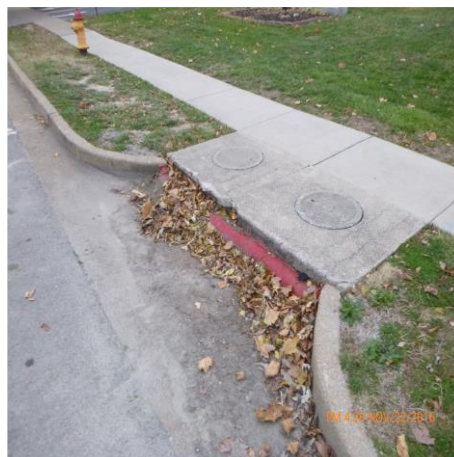
REMOVE SEDIMENT IN FRONT OF CURB INLET
