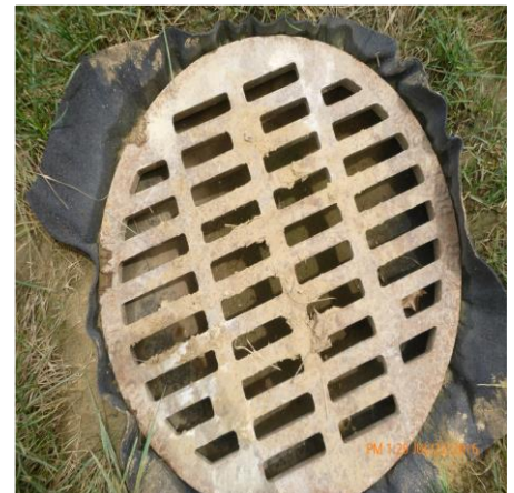
FILTER FABRIC IN PLACE AT INLET
