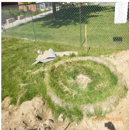
SILT SOCK AND FILTER FABRIC PROTECTING GI 23K2-0406D
