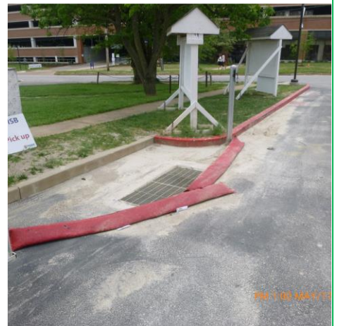
INLET PROTECTION IN PLACE
