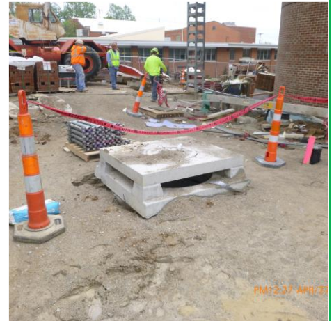
ADD PROTECTION TO AREA INLET # 4
