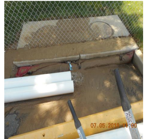
REMOVE SEDIMENT IN FRONT OF INLET PROTECTION
