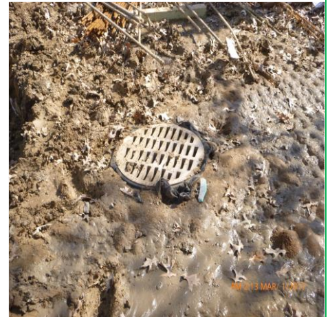
MONITOR SEDIMENT AT CURB INLET (PARKING LOT)
