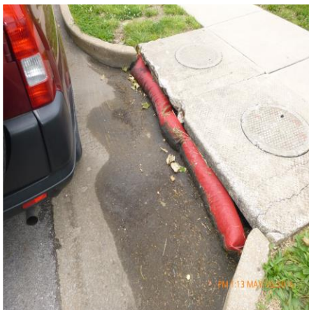
CURB INLET PROTECTION ON GARDEN AVENUE
