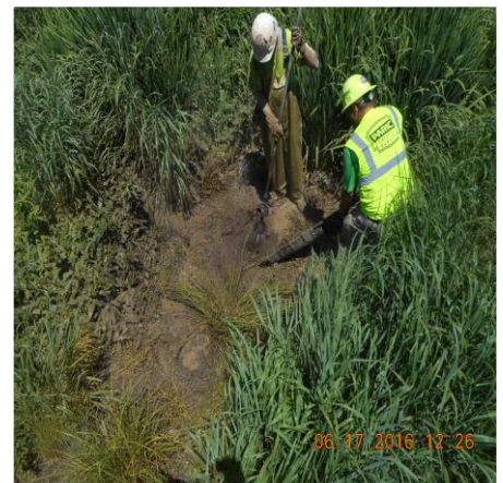
VIEW OF PRESSURIZED WATER AND VACUUMING OPERATION IN PROGRESS
