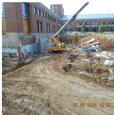
LOOKING SOUTH AT MIDDLE OF CONSTRUCTION SITE
