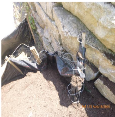
REINSTALL SILT FENCE
