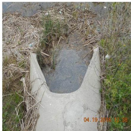
LOOKING AT EAST INLET PIPE INTO LAKE SOUTH OF PROJECT SITE
