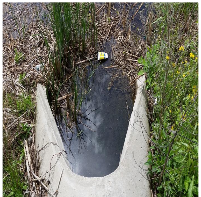
LOOKING AT CLEAR WATER STANDING IN INLET PIPE FES
