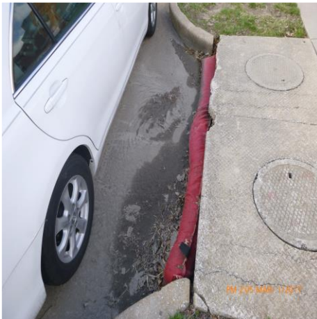
MONITOR SEDIMENT LEAVING SITE (PARKING LOT)
