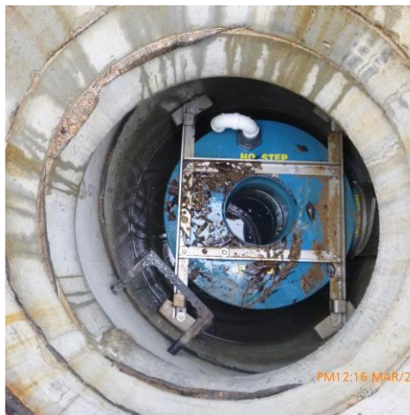
LOOKING AT INSIDE OF DOWNSTREAM DEFENDER
