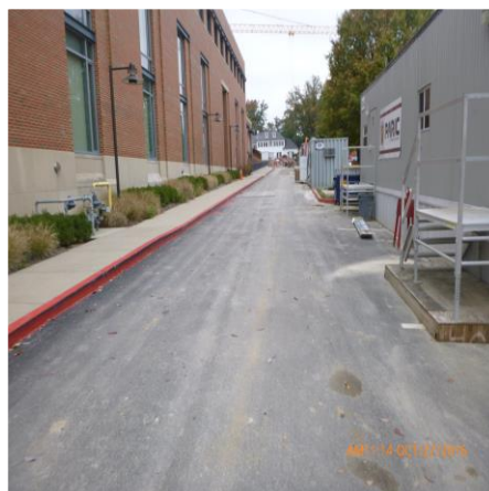
LOOKING NORTH AT CONSTRUCTION SITE ENTRANCE
