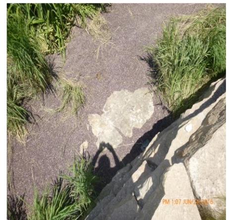
TEMPORARY REPAIRS TO BIODETENTION BASIN ARE COMPLETE
