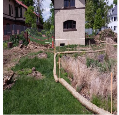
VIEW OF SEDIMENT PROTECTION AROUND EXISTING RAIN GARDEN
