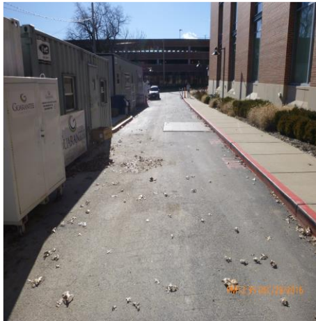
LOOKING AT SITE ENTRANCE FROM GARDEN AVENUE
