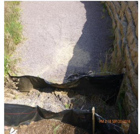
MONITOR SEDIMENT AT CONSTRUCTION SITE ENTRANCE BIG BEND
