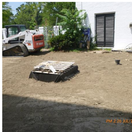
INLET PROTECTION IN PLACE
