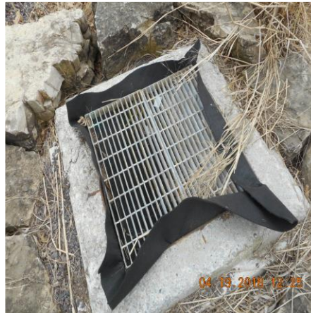
LOOKING AT SEDIMENT PROTECTION IN GI 23K2-0391D
