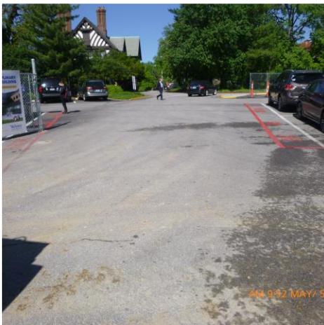
MONITOR SEDIMENT AT SITE ENTRANCE (PARKING LOT)
