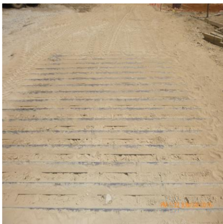
MONITOR CONDITION OF EXIT RAMP RUMBLE STRIP
