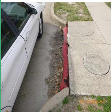
INLET PROTECTION IN PLACE (GARDEN AVENUE)
