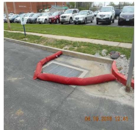
BIG RED INLET PROTECTION IN PLACE NEAR SOUTH END OF EAST DRIVE
