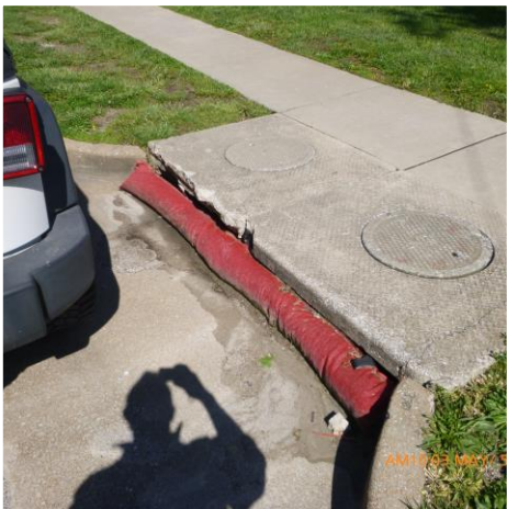
MONITOR SEDIMENT AT CURB INLET (GARDEN AVENUE)
