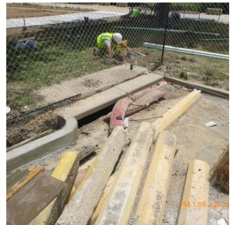
REPLACE SILT SOCK AND REMOVE SEDIMENT FROM INLET
