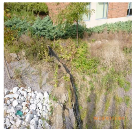
REINSTALL SILT FENCE UNTIL HILL HAS STABILIZED
