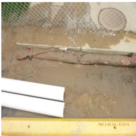
REMOVE SEDIMENT IN FRONT OF INLET PROTECTION
