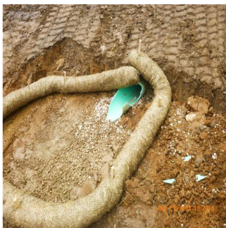
MONITOR SILT SOCK CONDITION AT EXISTING PVC PIPE AFTER EACH RAIN
