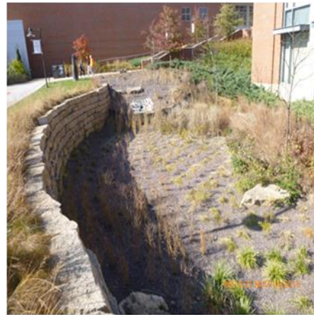
REMOVE SEDIMENT FROM IN FRONT OF CURB INLET
