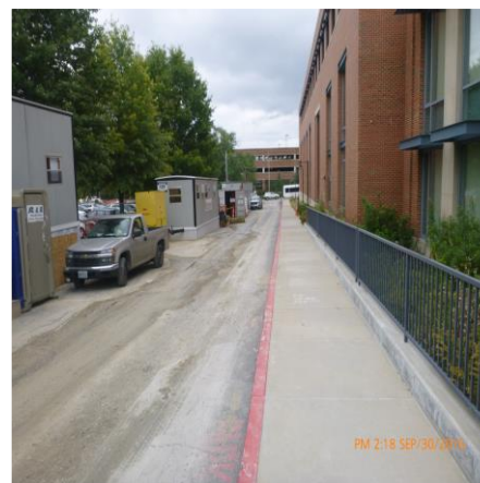
LOOKING SOUTH AT CONSTRUCTION DRIVEWAY ENTRANCE
