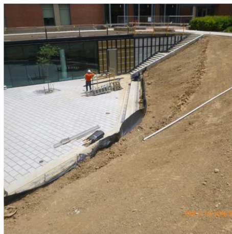
SILT FENCE INSTALLED ABOVE PATIO AREA
