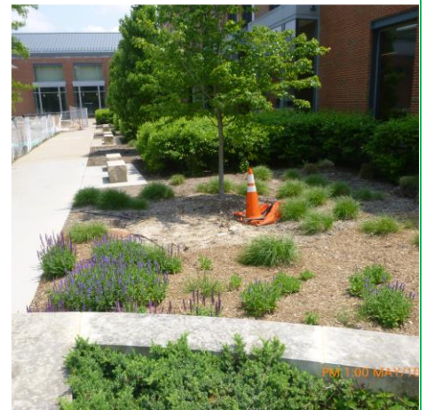
INLET PROTECTION IN PLACE
