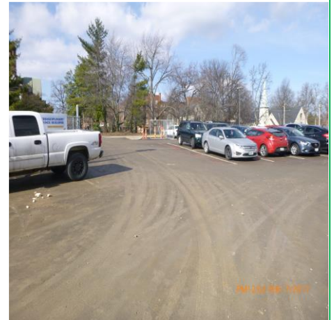
MONITOR SEDIMENT LEAVING SITE (PARKING LOT)
