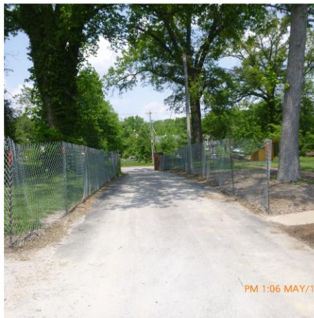
MONITOR SEDIMENT AT SITE ENTRANCE (BIG BEND ROAD)
