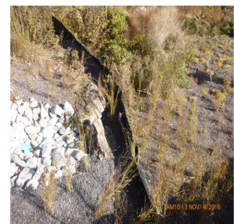
SILT FENCE IN PLACE IN RAIN GARDEN
