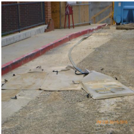
FILTER BAGS TO COLLECT SEDIMENT BEFORE DISCHARGING
