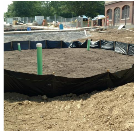
SILT FENCE IN PLACE AROUND RAIN GARDEN # 2
