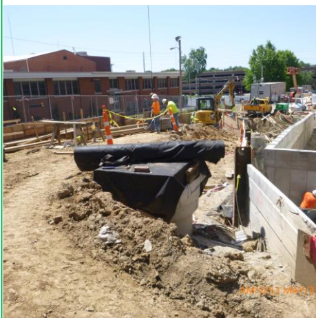
INLET PROTECTION IN PLACE
