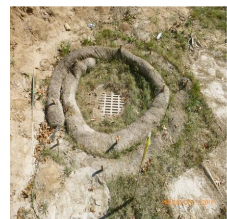
INLET PROTECTION IN PLACE
