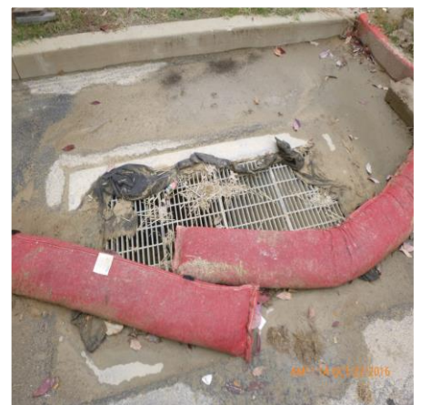
PIN OR WEIGH DOWN SILT SOCK, REPLACE FILTER FABRIC
