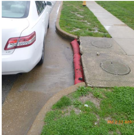
INLET PROTECTION IN PLACE (GARDEN AVENUE)
