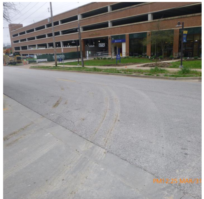
LOOKING EAST AT SITE ENTRANCE (GARDEN AVENUE)
