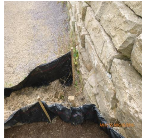
REINSTALL SILT FENCING BELOW DOWNSTREAM DEFENDER
