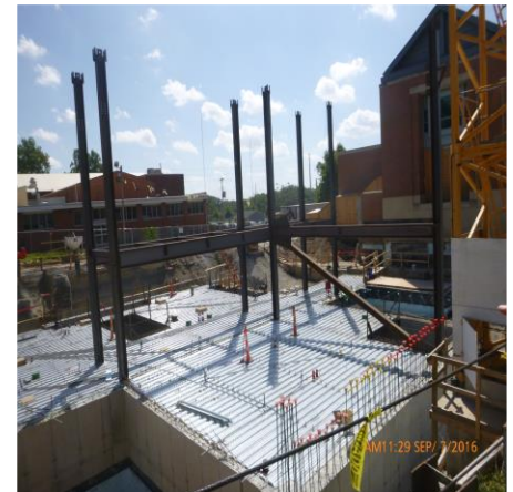
LOOKING SOUTH AT MIDDLE OF CONSTRUCTION SITE
