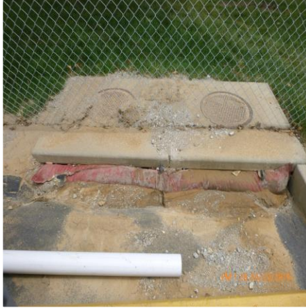
REMOVE SEDIMENT FROM IN FRONT OF INLET PROTECTION
