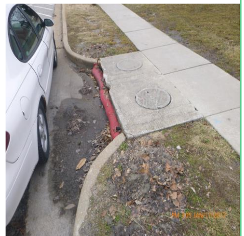
MONITOR SEDIMENT AT CURB INLET (GARDEN AVENUE)
