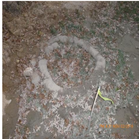
INLET PROTECTION IN PLACE
