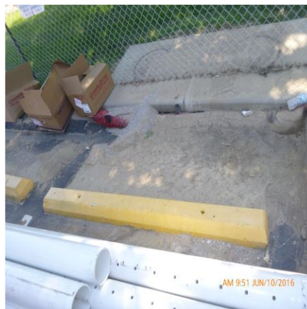
REMOVE SEDIMENT BUILDUP AT DCI 23K2-0374D
