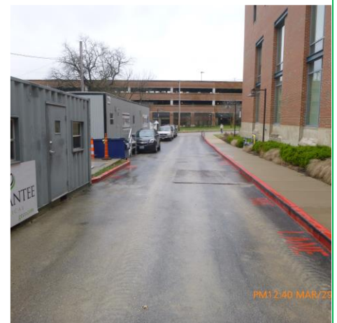
LOOKING SOUTH AT SITE ENTRANCE DRIVEWAY
