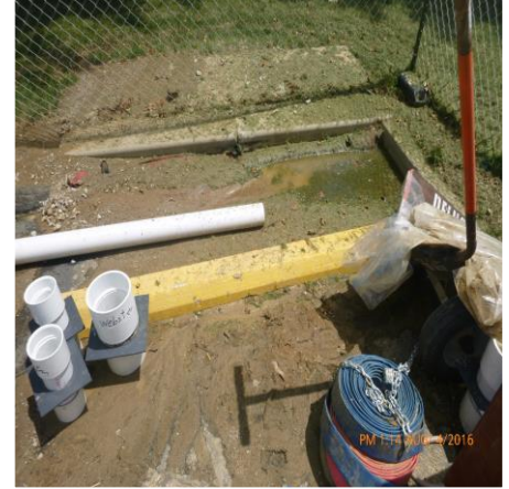
REMOVE SEDIMENT AROUND CURB INLET
