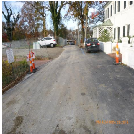
MONITOR SEDIMENT AT SITE ENTRANCE
