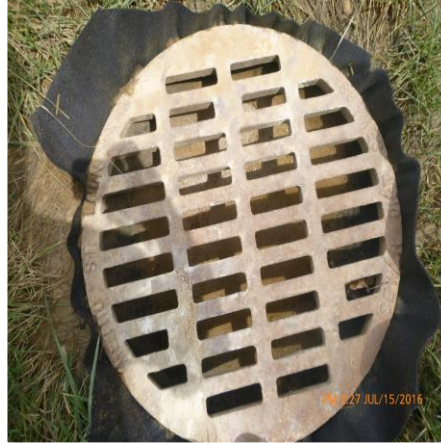
FILTER FABRIC IN PLACE AT INLET
