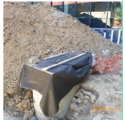
INLET PROTECTION IN PLACE
