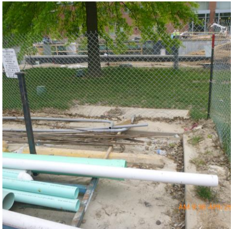
REMOVE SEDIMENT FROM IN FRONT OF CURB INLET (PARKING LOT)
