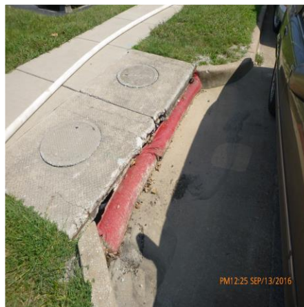
INLET PROTECTION IN PLACE (GARDEN AVENUE)
