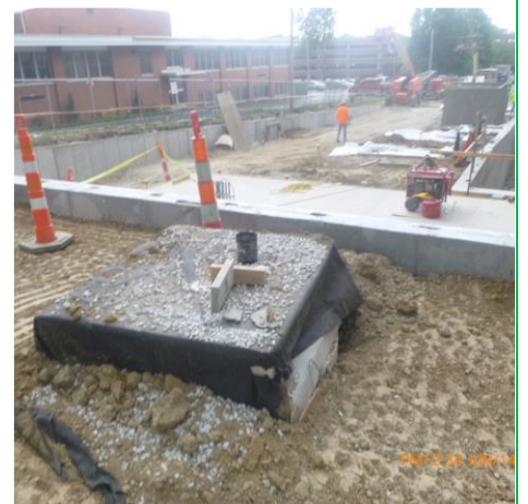
INLET PROTECTION IN PLACE
