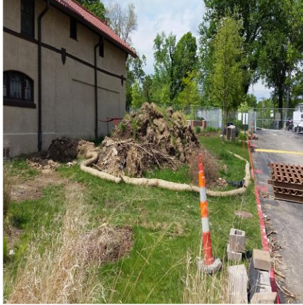
VIEW OF SEDIMENT BARRIER AROUND SOIL STOCKPILE
