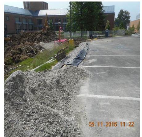
LOOKING SOUTH AT DIVERSION BERM ON WEST PARKING LOT
