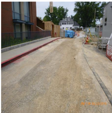
MONITOR SEDIMENT AT CONSTRUCTION DRIVEWAY ENTRANCE
