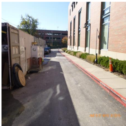
LOOKING SOUTH AT CONSTRUCTION SITE ENTRANCE
