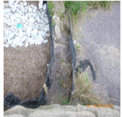
REINSTALL LOWER PORTION OF SILT FENCE
