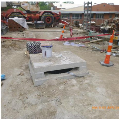
ADD PROTECTION TO AREA INLET # 4
