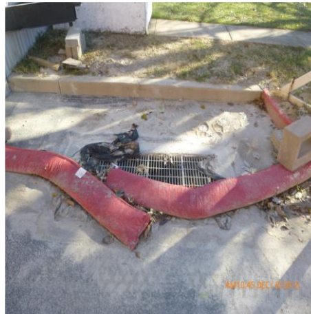
REPLACE FILTER FABRIC AS NEEDED
