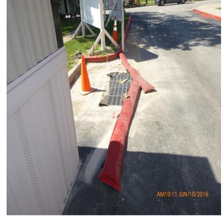
PIN OR WEIGH DOWN INLET PROTECTION 23K2-0394D
