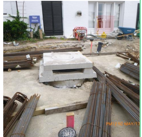
ADD PROTECTION TO AREA INLET # 4
