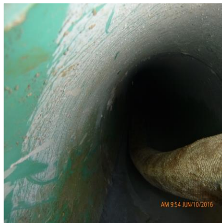
WATER PUMPED THROUGH HOSE INTO END OF PIPE
