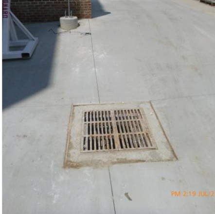
VIEW OF DBL GRATE INLET # 1 PROTECTED BY FILTER INSERT
